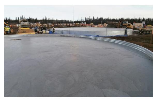
The use of corrugated steel panels is an effective and cost-saving technique for the construction of gravel filled or concrete filled foundation rings
